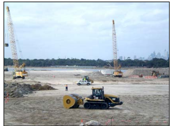
Figure 9a: HEIC process post Dynamic Compaction improvement at Port Botany.
