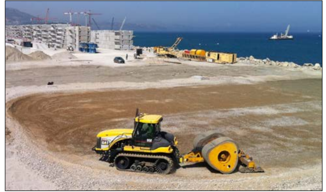
Figure 2a: 3-Sided 25kJ Landpac HEIC working on dredged marine sands in Morocco
